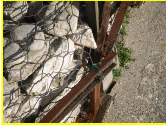
Patched repair of gabion (Asset Ref No. 1231D901D3201C03)
