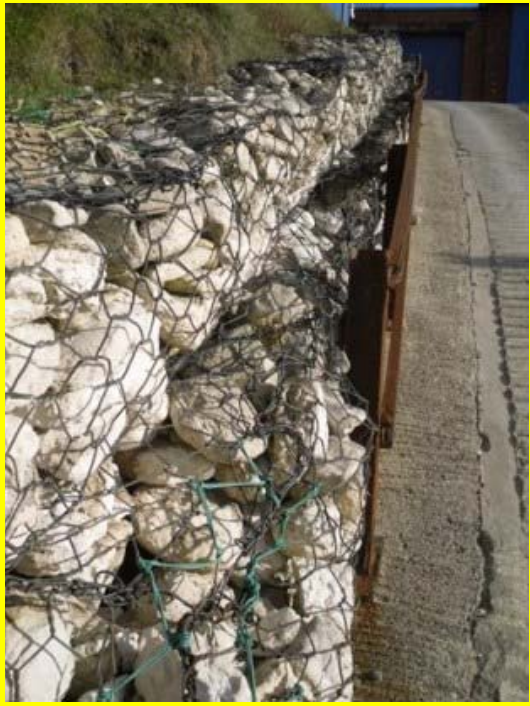
Overview of gabions and patched repair (Asset Ref No. 1231D901D3201C03)
