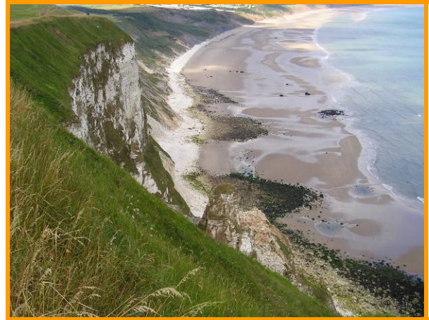
E108/2 recent rockfall and collapse of chalk pillar (Partly Active) (Note: this unit was previously classified as Locally Active in 2008)
