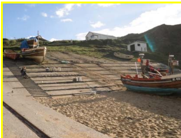
Slipway and revetment at North Landing (Asset Ref No. 1231D901D3201C02)
